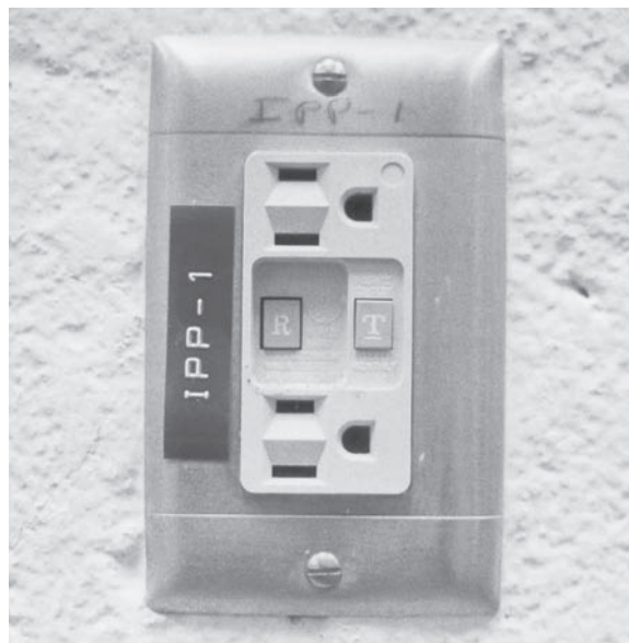
Figure 5-36 A typical ground-fault interrupter (GFI).
