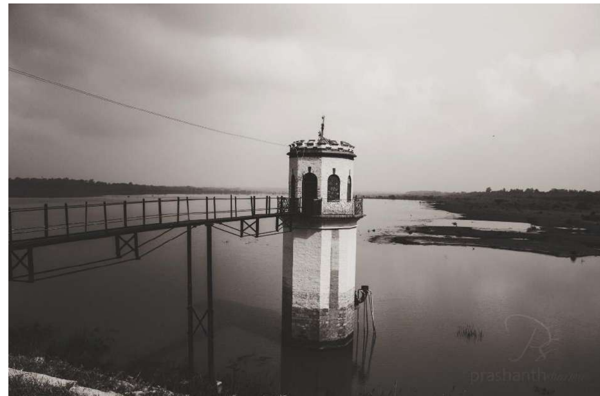
Pump house at Hessarghatta Lake
