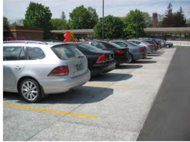
POROUS CONCRETE PARKING SPACES
