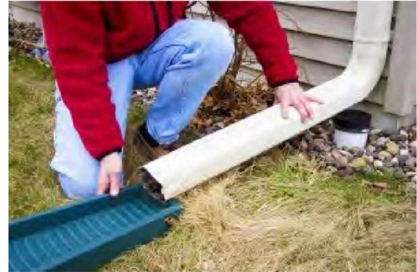
ONE FORM OF DOWNSPOUT DISCONNECTION
