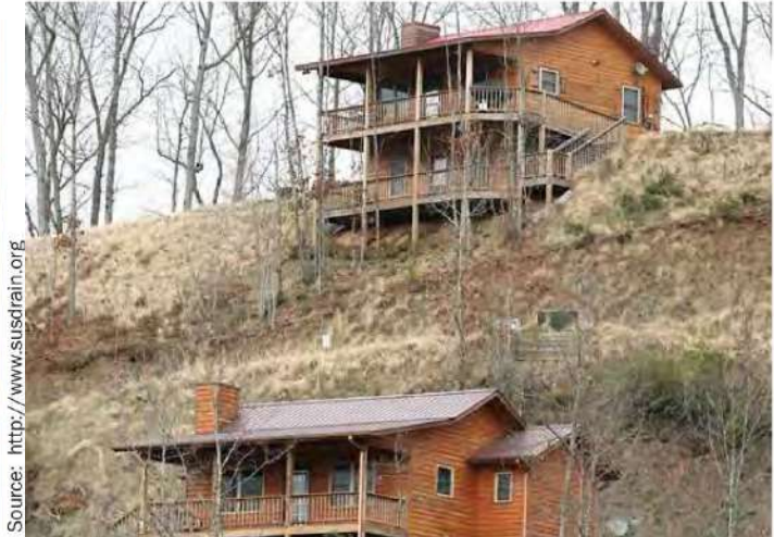
ALTERED HYDROLOGY ON A STEEP SLOPE
