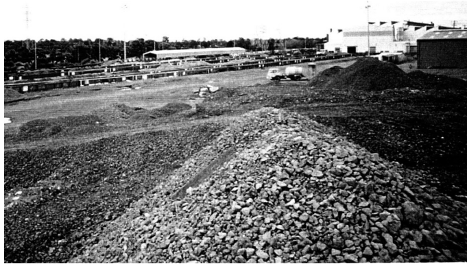
Figure 14.7 Stockpiles of waste ballast at Chullora (NSW).
