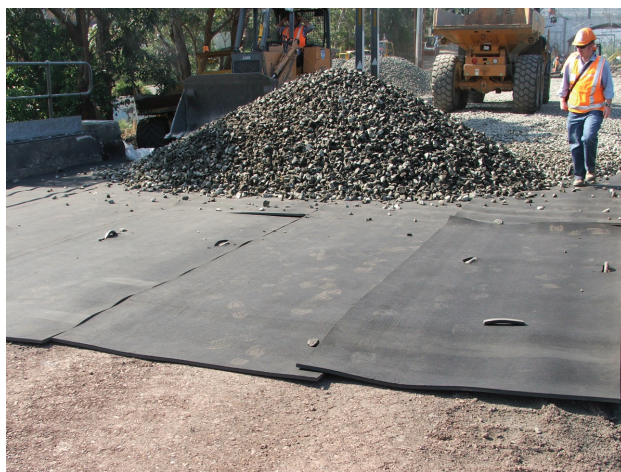
Figure C2 Placing of ballast mat over a bridge deck at Bulli.
