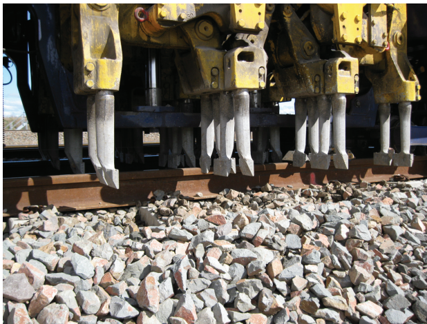
Figure C4 Automated tamping equipment at Singleton.
