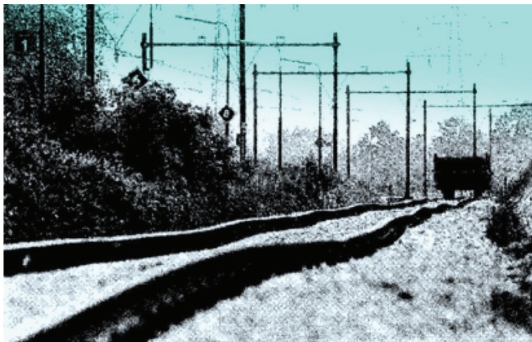
Figure 1.3 Differential settlement in rail track causing significant risk to trains (after Suiker, [9]).
