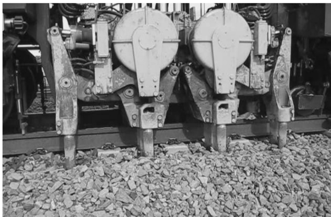
Figure 14.3 Tamping tines penetrating the ballast layer.
