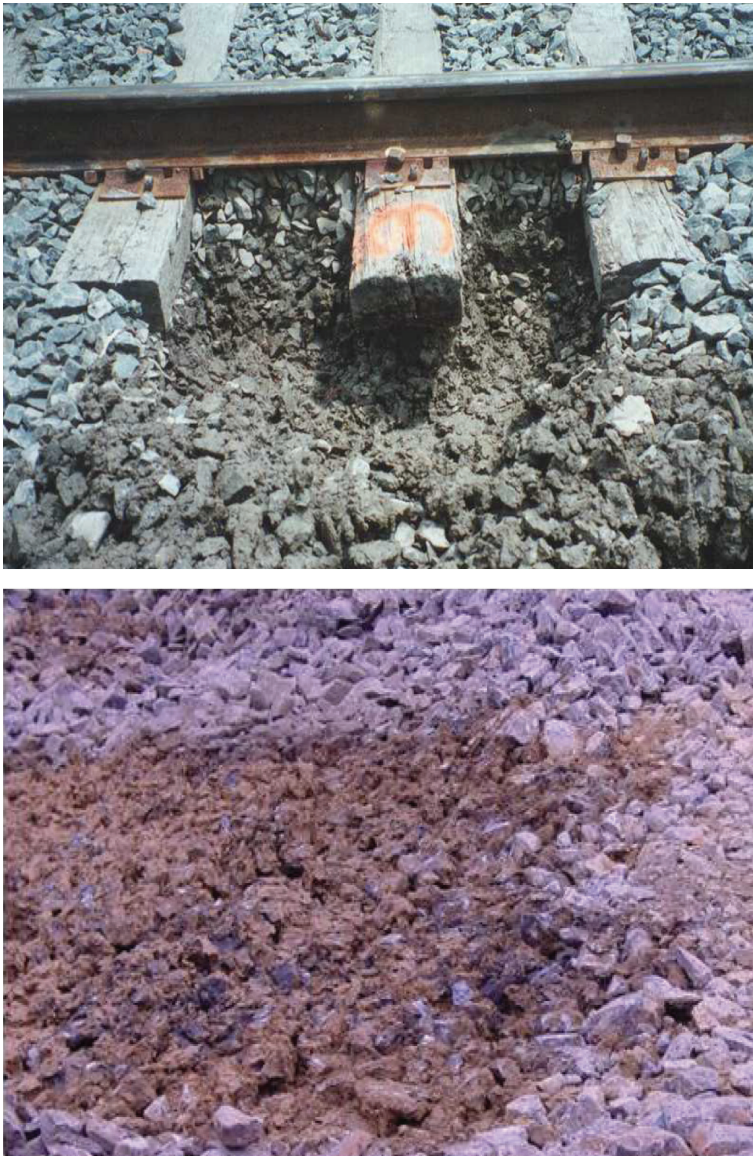
Figure 1.4 Fouled ballast.
