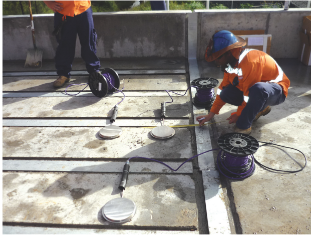
Figure C5 Installation of pressure cells at Mudies Creek bridge near Singleton.
