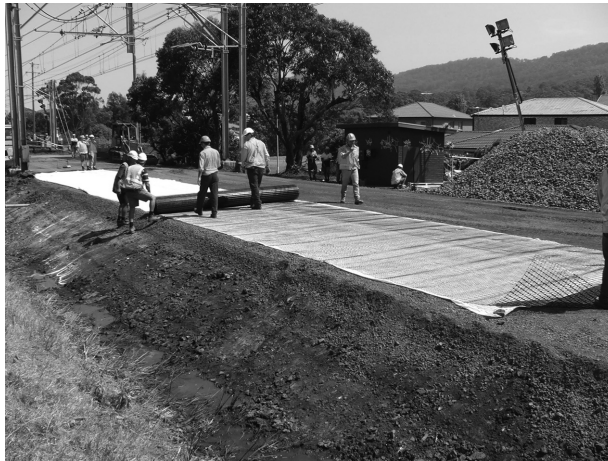
Figure 10.3 Placement of geocomposite over capping layer.
