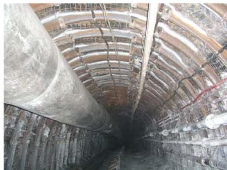
Figure 7. Roadway at Bogdanka mine with arches back-filled with binding material.
