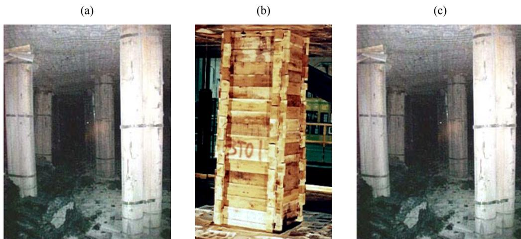
Figure 3. Selected types of standing support being applied in gateroads in the U.S.; Can support (a), Link-N-Lock crib (b), Cluster Props support (c).
