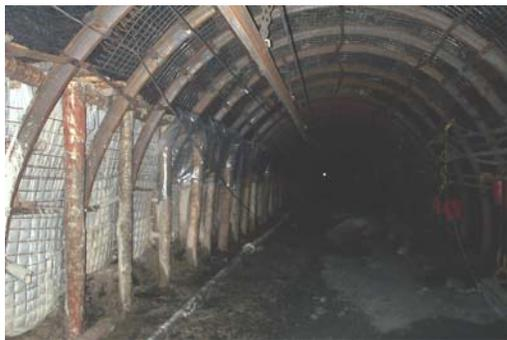
Figure 6. Reinforcement of steel yielding arches in gateroads by means of: (a) bolting cross bar arches with fully resin steel bolts, (b) roadside pack of mineral binding material.
