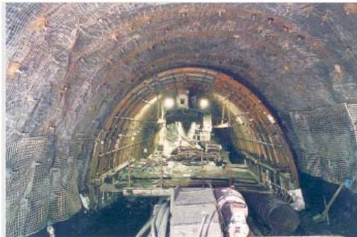
Figure 5. Working development in combined support, type A (Eikhoff 2009).
