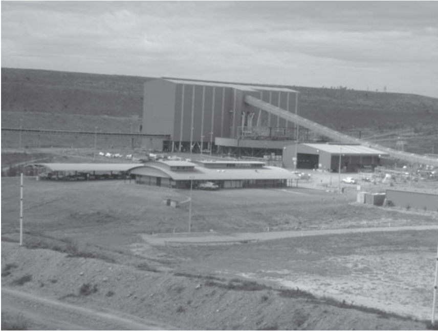
Figure 2.27 Clean industrial operations: Enclosures to protect against Noise & Dust. 30
