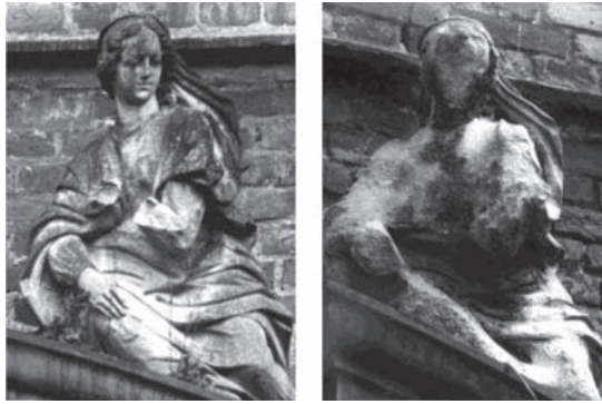
Figure 3.9 Effects of Acid Rain to materials/rocks. Deterioration in the shape of Sandstone figure over the portal of a castle in Westphalia, Germany due to acid rain. 18
