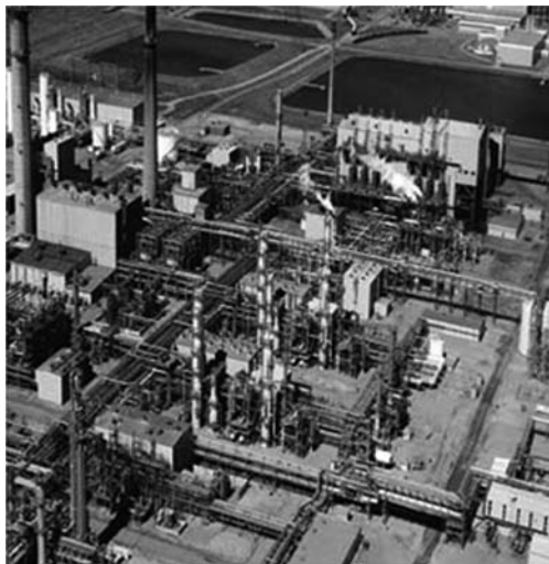
Figure 12. CO 2 precombustion capture at a coal gasification plant in North Dakota (IPCC, 2011).
