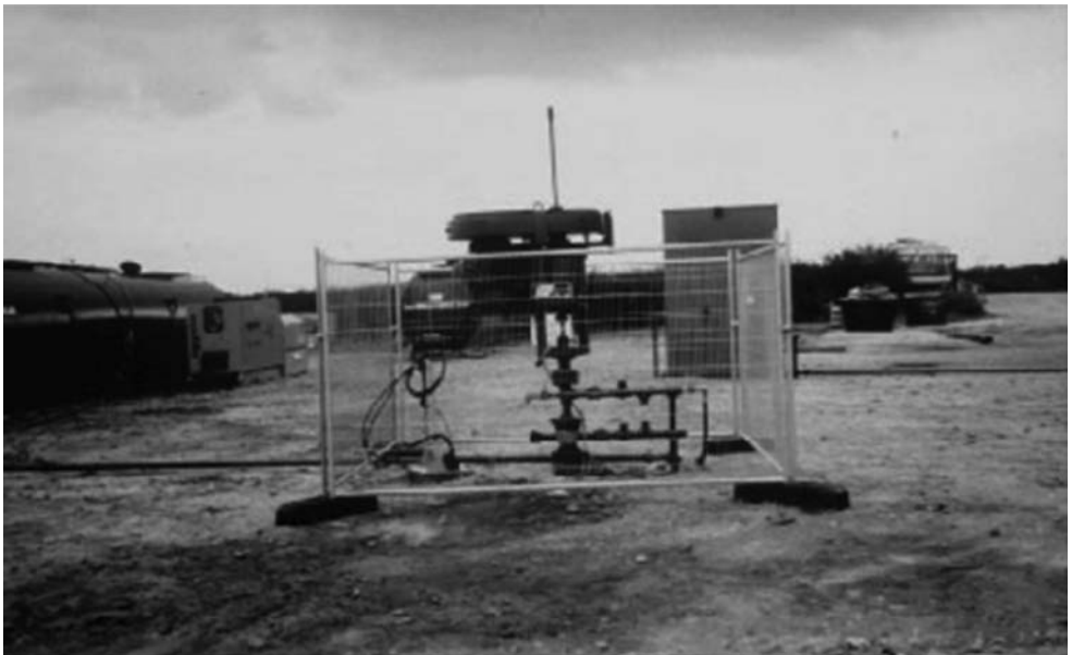
Figure 32. Coal bed methane test well at Sealand, Chester, UK (Evergreen Resources).
