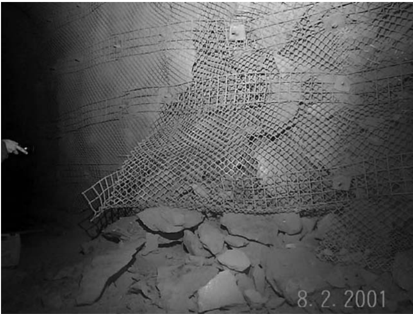
Figure 18.3 A fault-slip rockburst in a deep metal mine (Simser, 2001).
