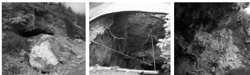
Figure 15.65 Caving or damage to natural caves in L'Aquila earthquake.
