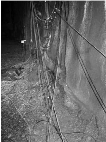
Slot tunnel showing soil movement after Test #3
