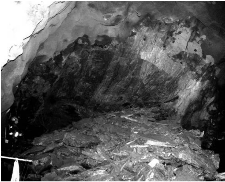
Figure 18.1 Rock pieces that burst down from the roof in a deep metal mine.
