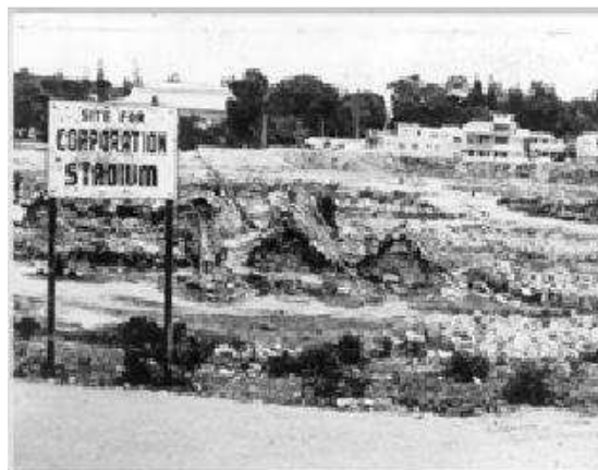
Figure 9: Sampan Sampangi Tank bed for Stadium Construction. (Ref. www.cscsarchive.org ).
