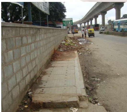
Fig. 4: The walkway under investigation.
